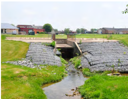
Stormwater device at Rockvale Outlet
