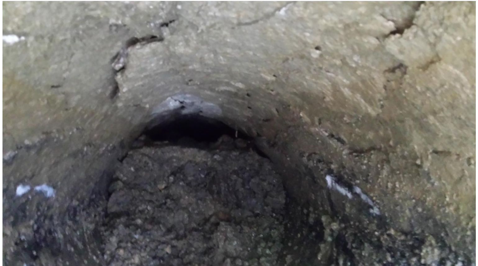
Degraded interior of sewer line which collapsed parallel to Tennyson Ave.
