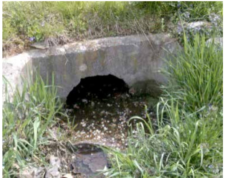
Figure 2: Sediment buildup
